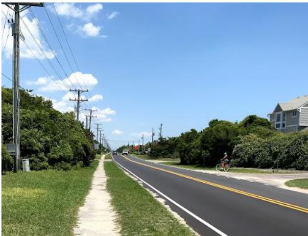
Figure 3.7: Four-foot sidepath and cyclist attempting to cross NC 50.
